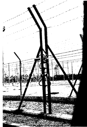
Fence protection system.
